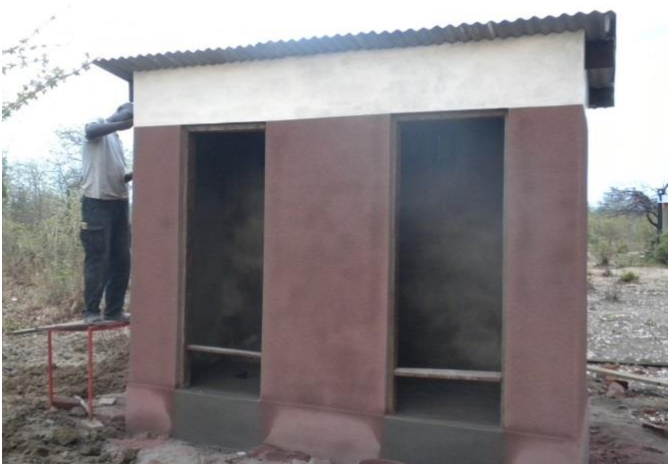
Toilet/Bathroom under construction
