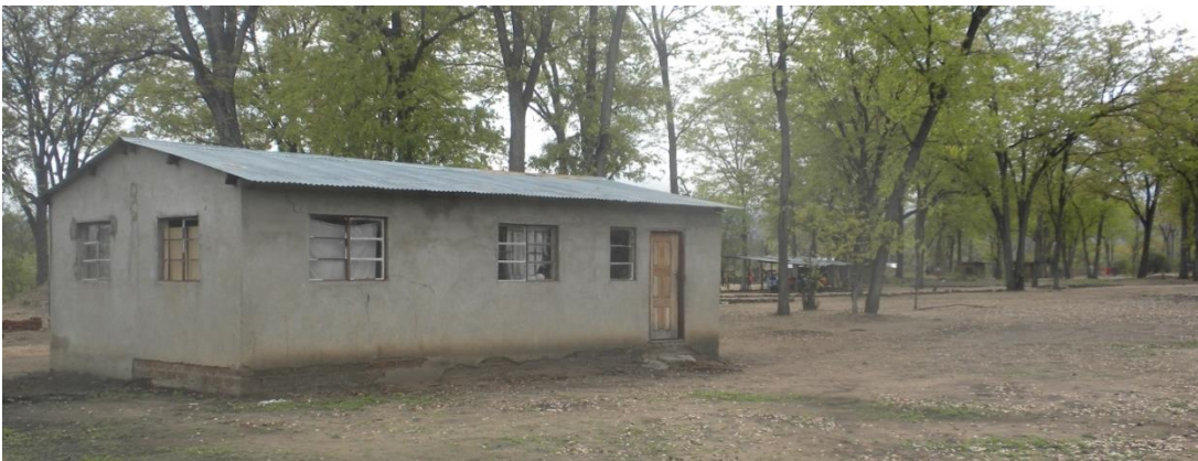
The house having its roof fixed
