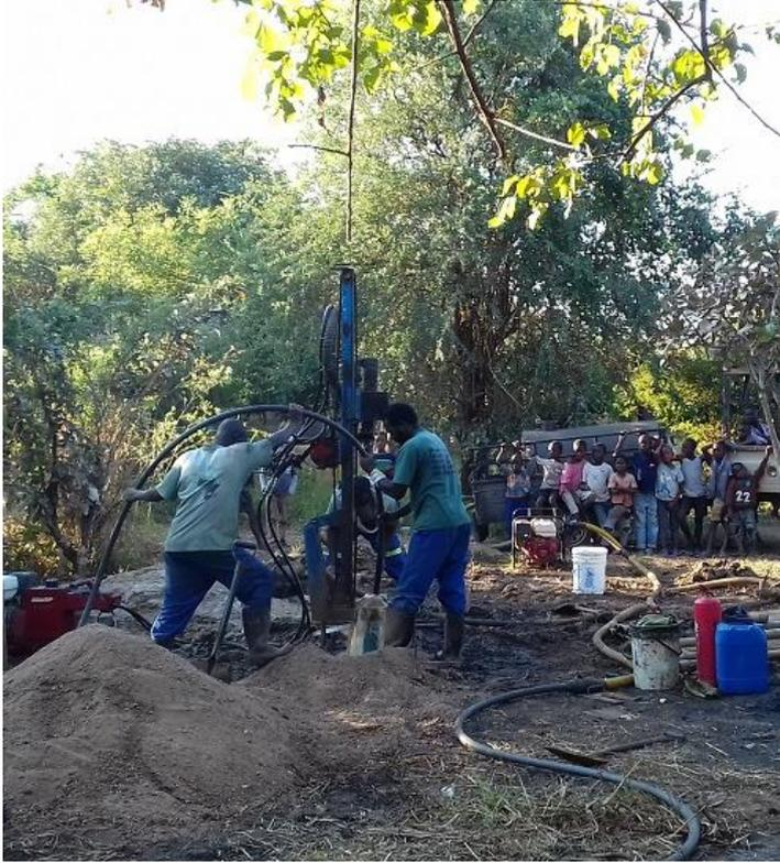
Drilling finished, casing in – installing the gravel pack filter.
