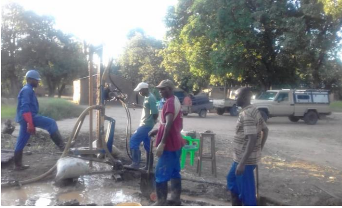
Drilling underway at Chikosi Village
