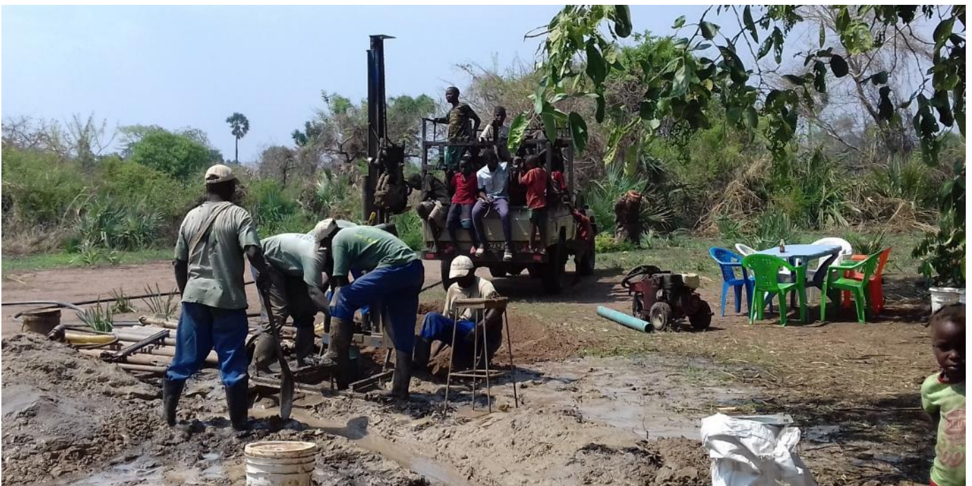
Drilling underway at Sapulani
