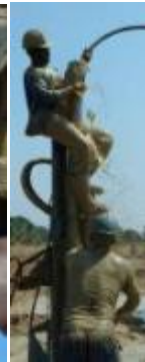
Putting in the casing, flushing out the borehole and pump testing – lots of good clean water.
