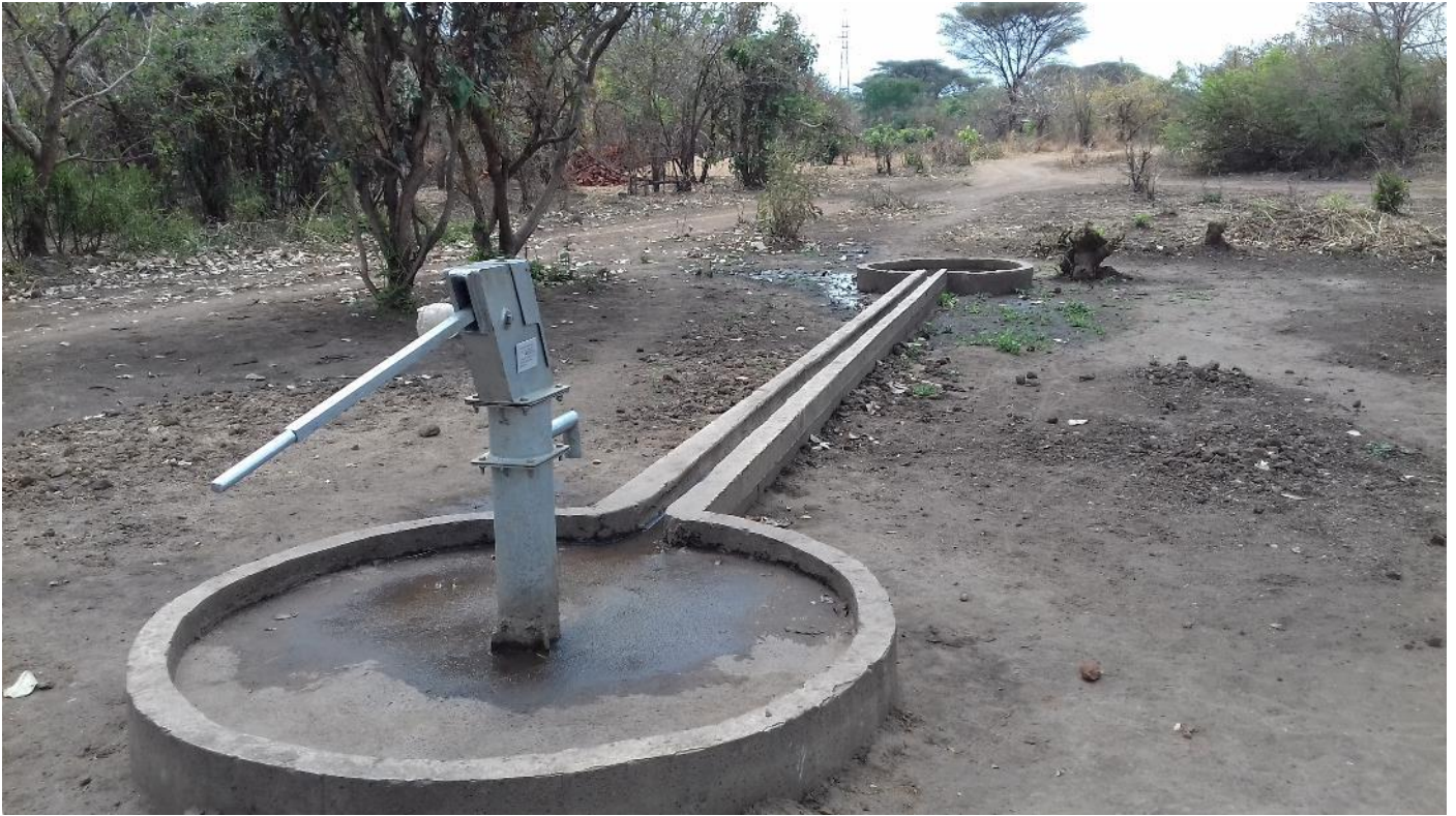
The finished Mwezi Village borehole
