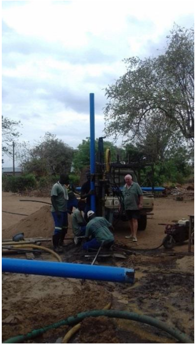
Installing the casing
