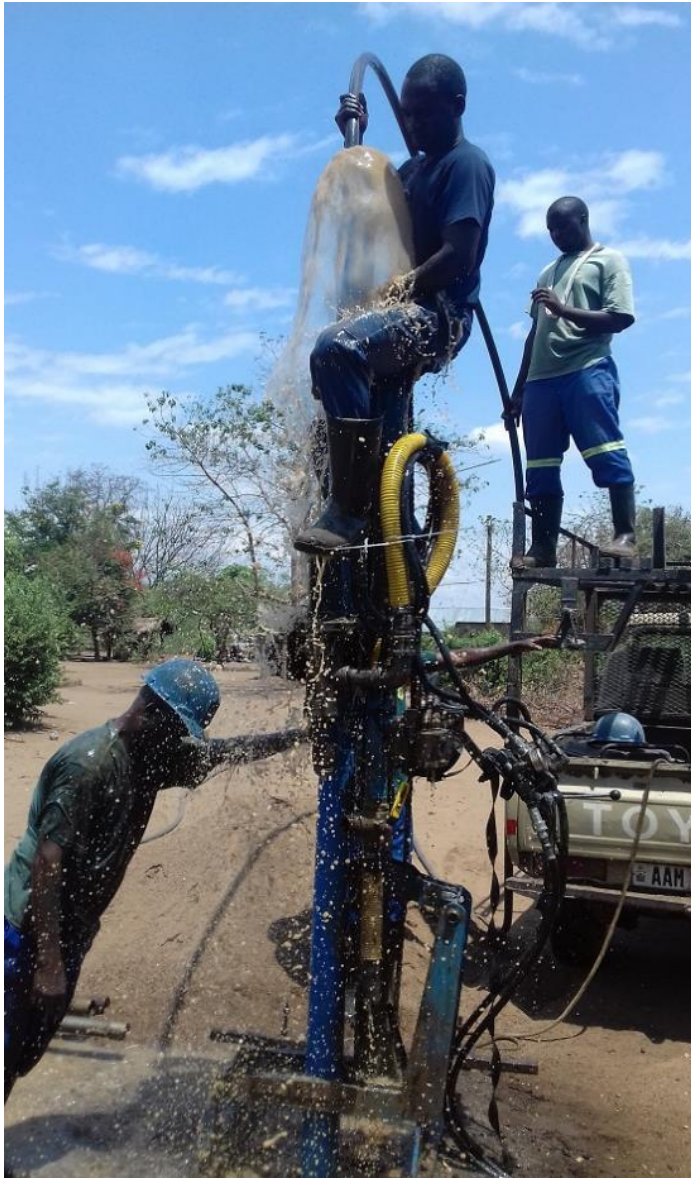
Drilling in action
