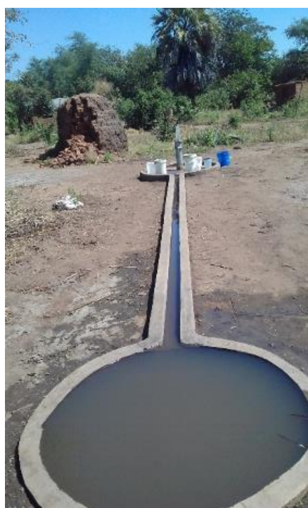
New village borehole
