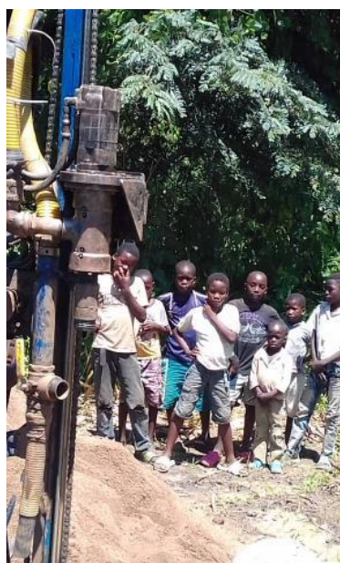
Local children watching the drilling with interest.
