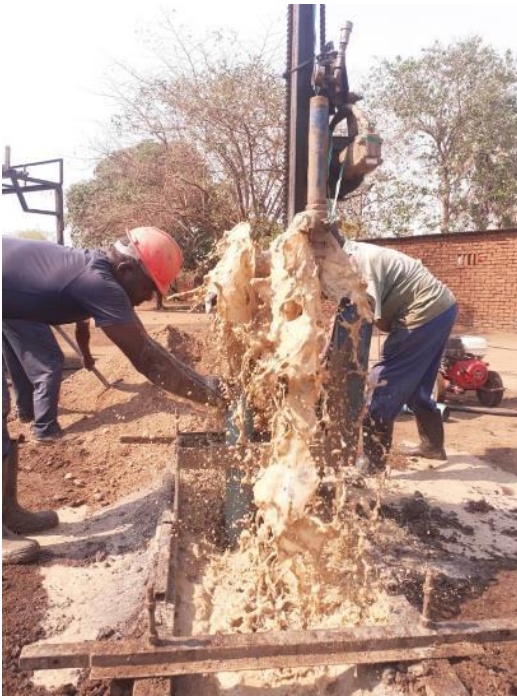
Putting in the casing at Kalumba.
