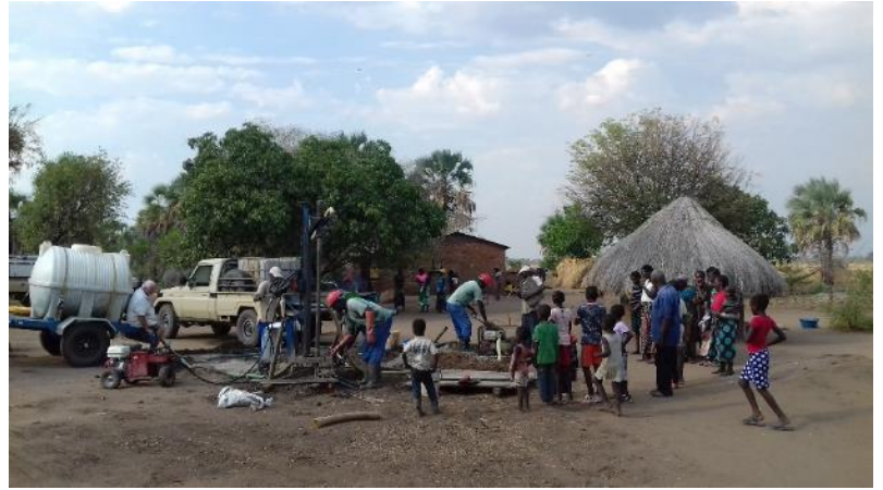
Drilling underway at Kalumba Village
