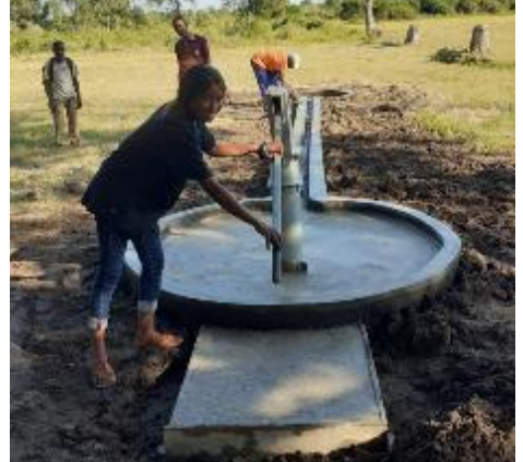
Trying the new pump
