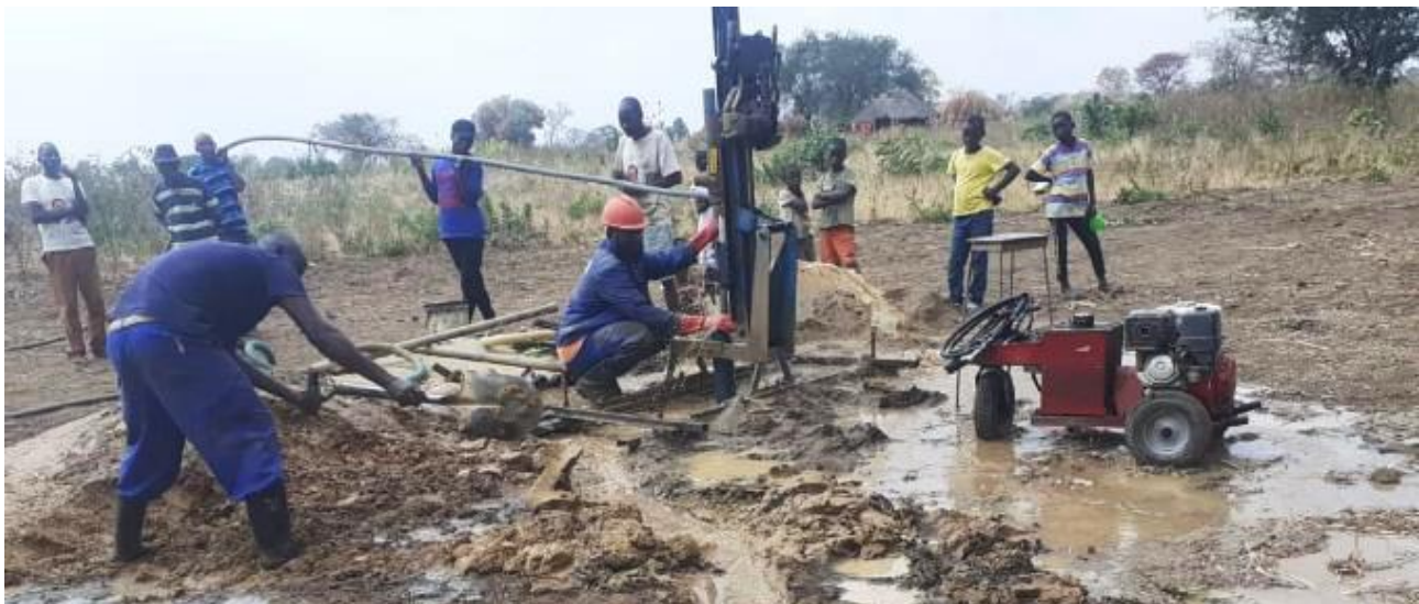
Drilling underway at Malanda
