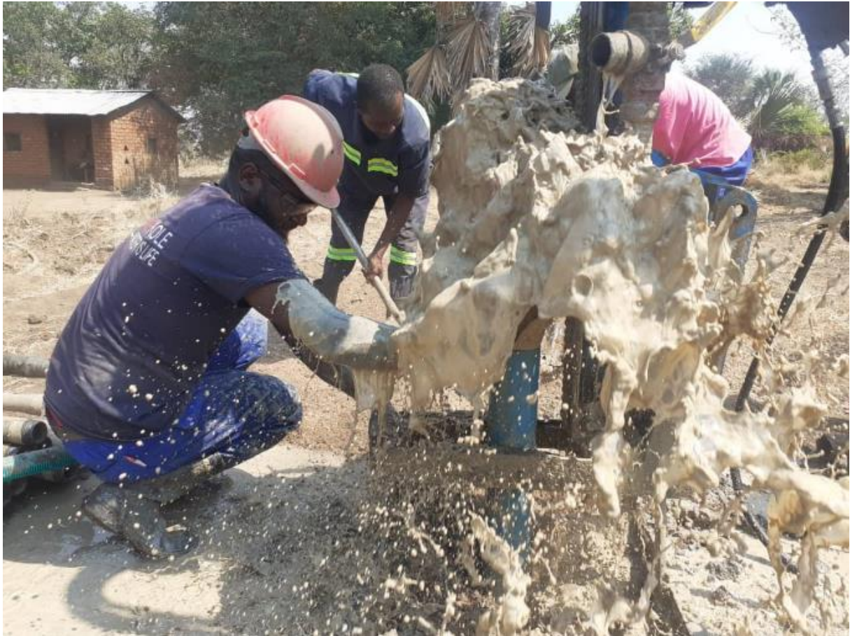
Drilling underway at Mazikila
