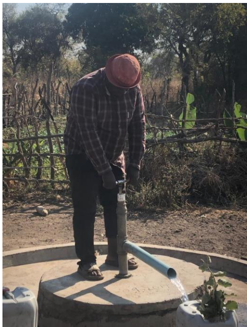
Well capped and small pump installed - not enough capacity meaning a very long wait from before light for women water collectors. Capped wells are unhygienic and most only function for 7 months per year.
